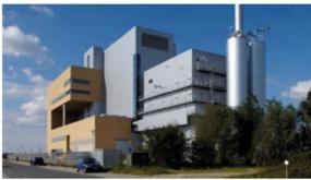
Paper production consumes a lot of energy, in order to meet the plant's demand refuse-derived fuel (RDF) power plant was established. For more than a decade, the thermal energy required for paper drying has been supplied by the RDF run plant. Refuse-derived fuel is procured locally which helped reduce the transport costs and CO2 emissions.
